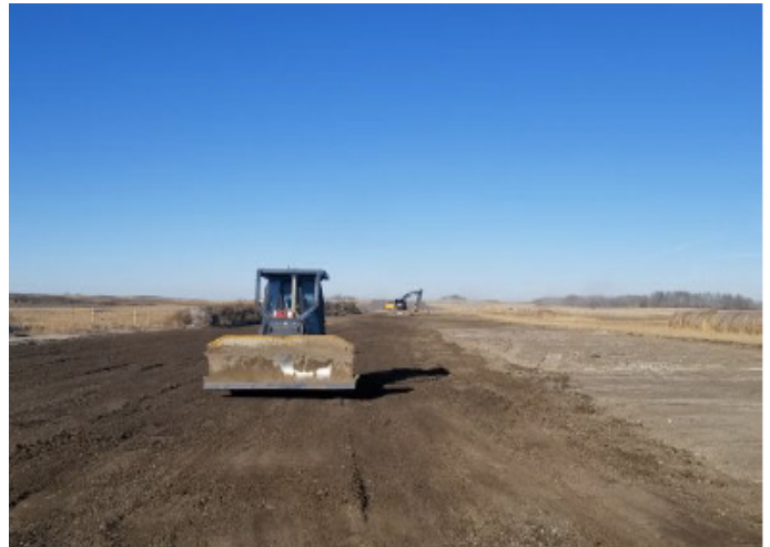
Levelling the ROW – SF 62 - Oct 22, 2018
