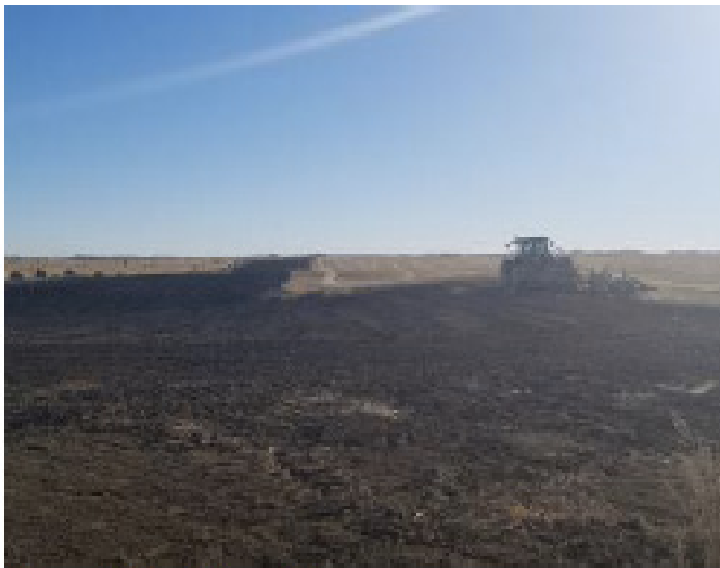
Tractor ripping topsoil for decompaction - SF 56 - Oct 26, 2018
