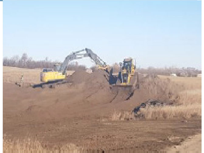
Excavator and dozer moving topsoil back - SF 79 - Oct 27, 2018
