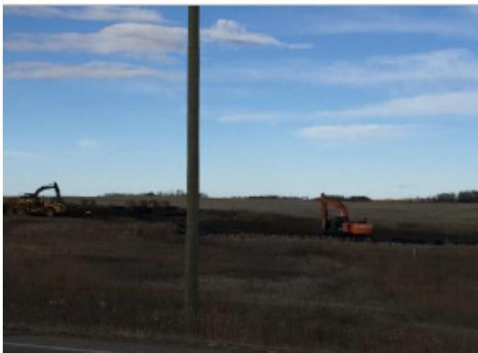
Wetland ramp removal - SF 44 - Oct 27, 2018
