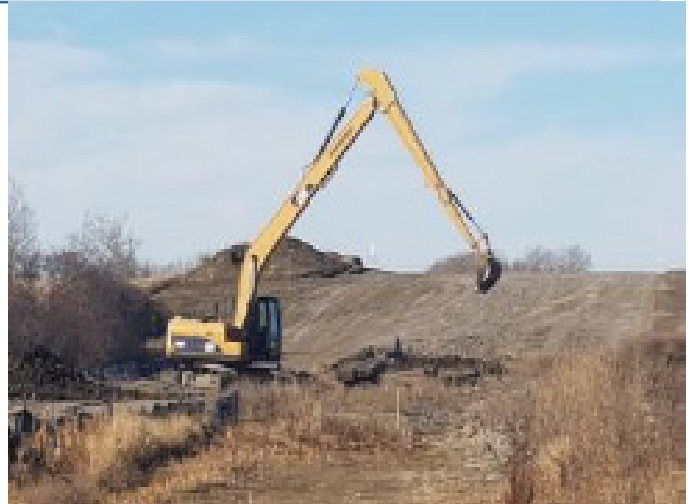
Excavator ramp removal - SF 51 - Oct 26, 2018
