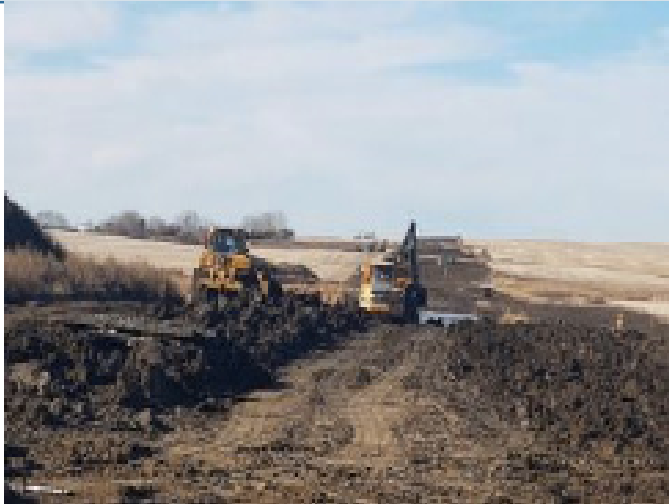
Ramp removal - SF 50 - Oct 26, 2018
