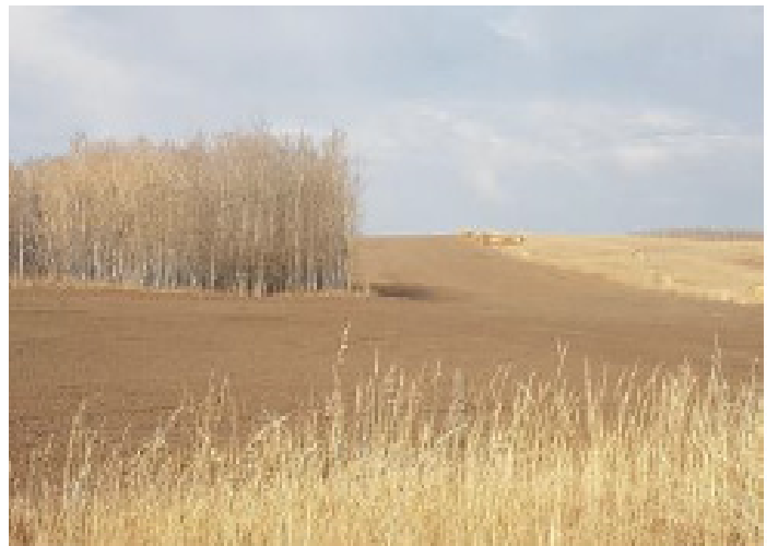
ROW covered and completed with topsoil - Oct 25, 2018
