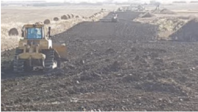
Dozer spreading out transition – SF 49– Oct 22, 2018
