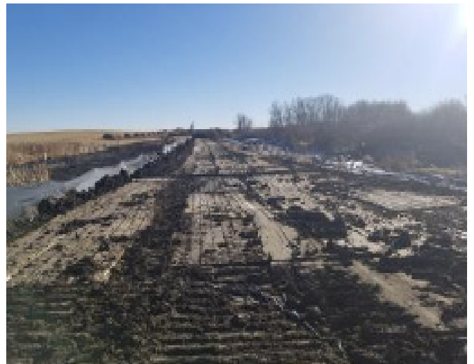
Stripping material off of wetland matting - SF 52 - Oct 26, 2018
