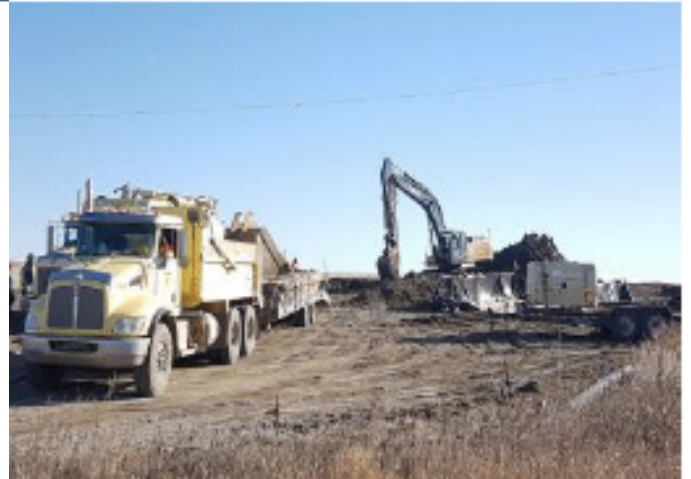
Crew working on ovality dig – SF 65 - Oct 23, 2018
