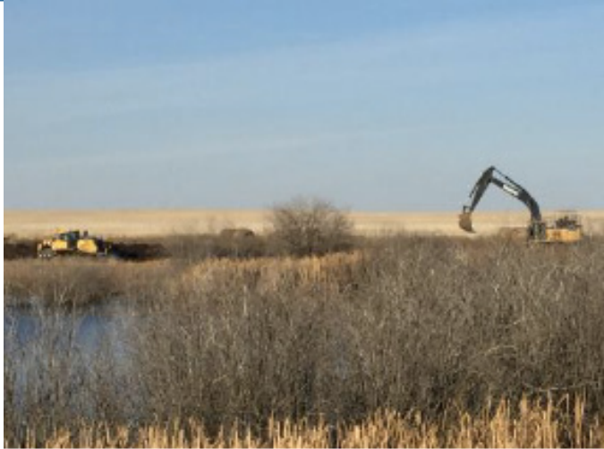
Excavator working on wetland– SF 49 – Oct 24, 2018
