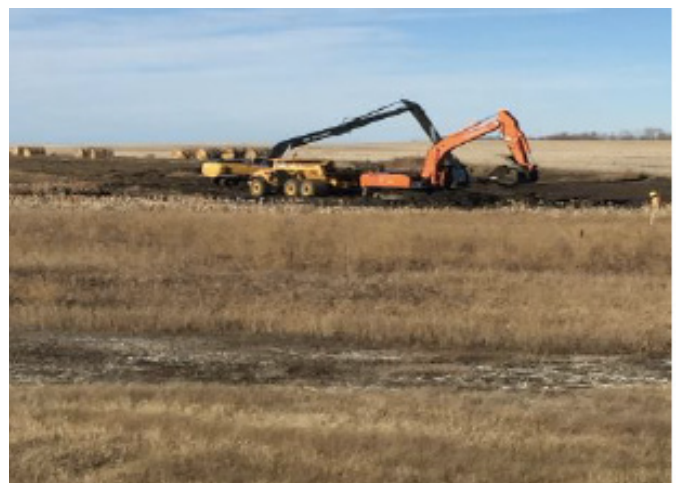
Ramp removal - SF 44 - Oct 26, 2018
